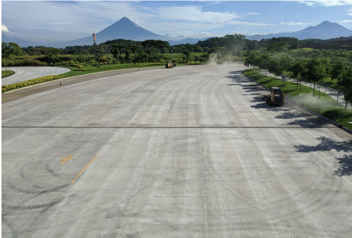
Michatoya Pacifico, still under construction.
